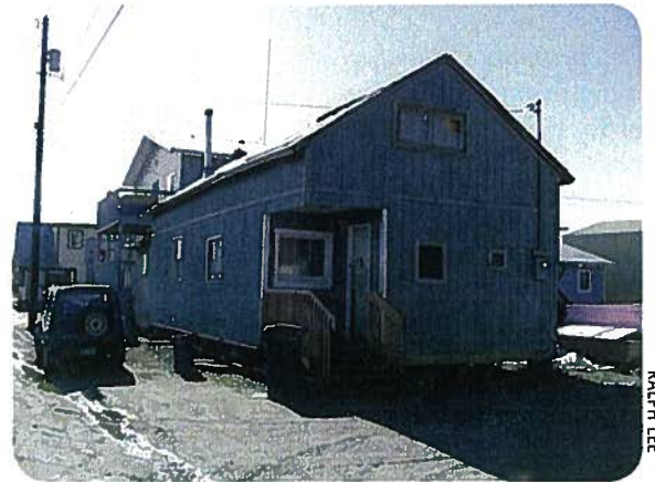
This is an "after" photo of a home in Nome, a joint weatherization/rehab project that included the Nome Eskimo community and the United States Department of Agriculture Rural Development program.
