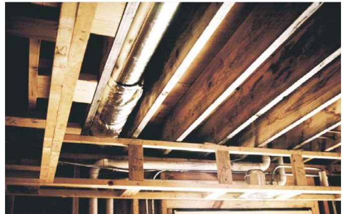
Photograph 4: Soffit on Exterior Wall —Wow, this allows for connecting your entire floor cavity to the outside.
