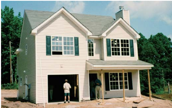
Photograph 10: Bedroom Over Garage —Unfortunately, in my experience, garages are not effectively isolated from houses, especially at the second floor assembly to interior garage perimeter.
