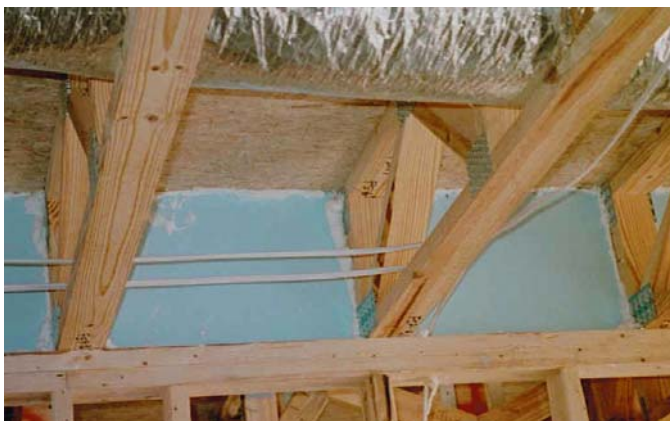
Photograph 11: Bedroom Over Garage Done Well —Notice how beautifully the floor joists are draftstopped over the top of the wall that separates the interior garage perimeter from the house. This location typically represents a huge leakage area (aka, big holes).
