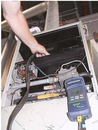
70+ Furnace: Sample flue gases in the draft diverter. Measure draft in the vent connector above the furnace.
